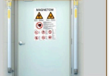
Cloud Magnet Ferro Detector
